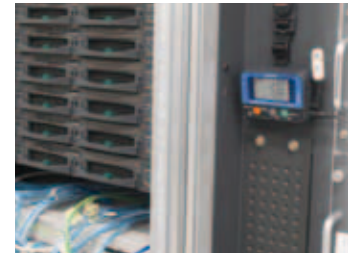
Recording temperature and humidity in a server room
